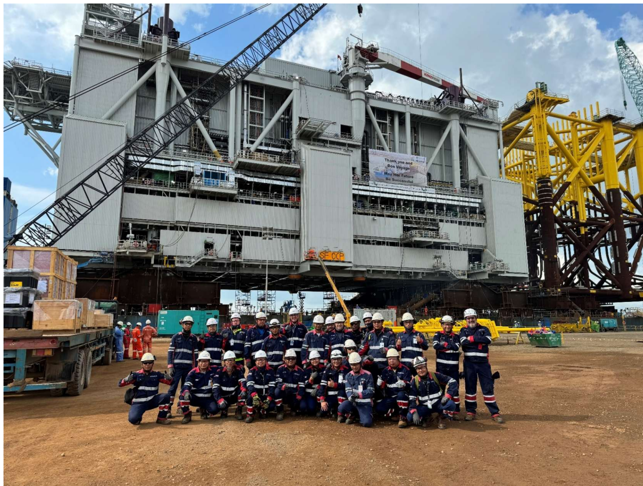
Offshore converter topside and jacket load-out July 2024
