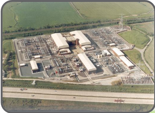
Sellindge IFA Substation
