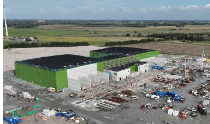
A-Nord 2GW VSC HVDC construction
