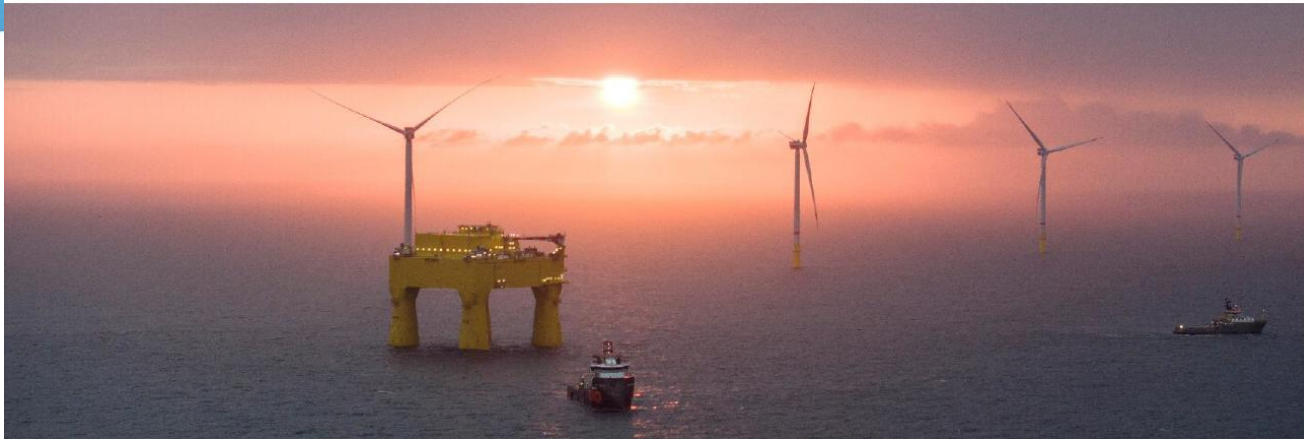
Dolwin Epsilon commissioning
