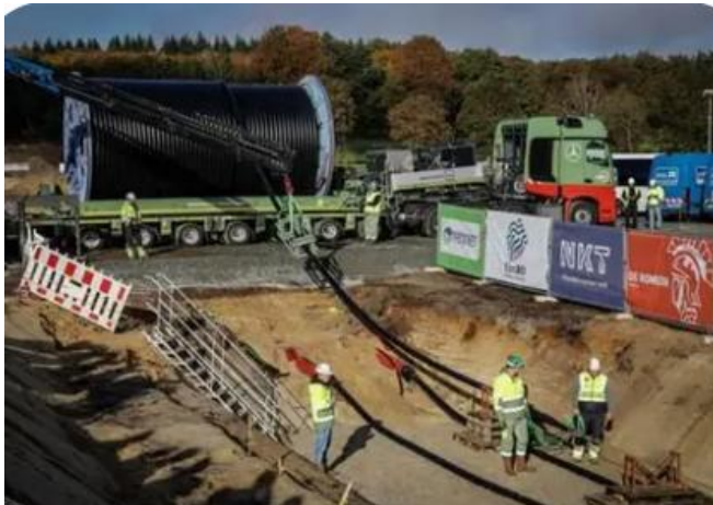
Cable installation on Suedlink
