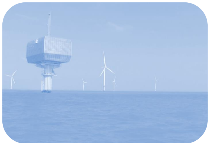
Connecting OSW at Distance
