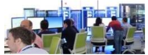
Control Room at The National HVDC Centre
