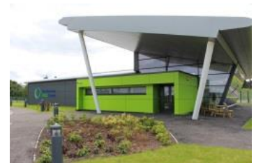
The National HVDC Centre
