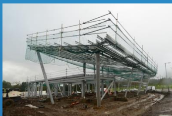
View of the Main Entrance
